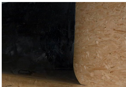
Buffer protection in the pellet depot
